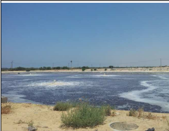
Khanyounis Wastewater Treatment Plant
